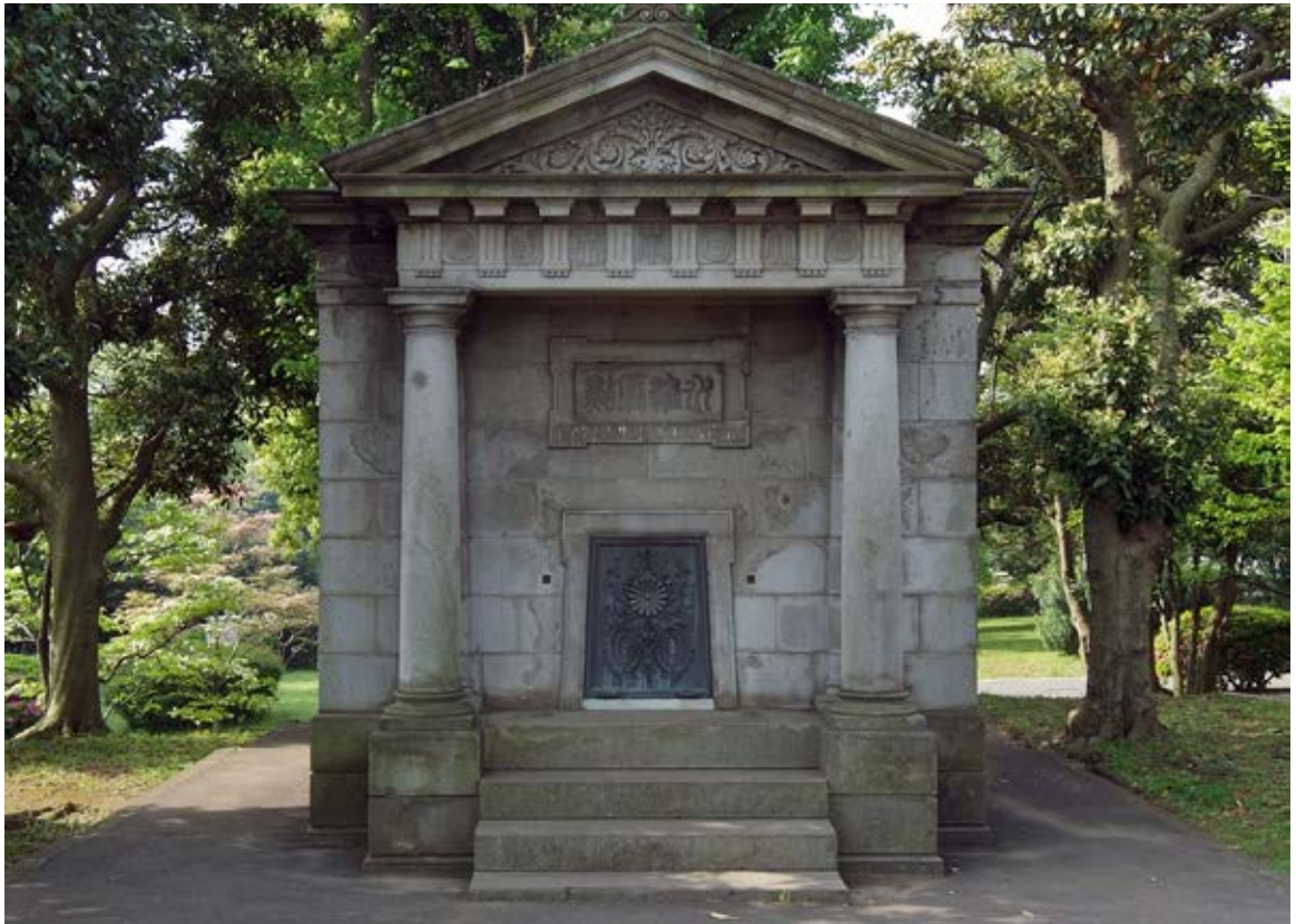
Figure 48 The Japan Standard building in Tokyo (Wiiii, n.d.)
